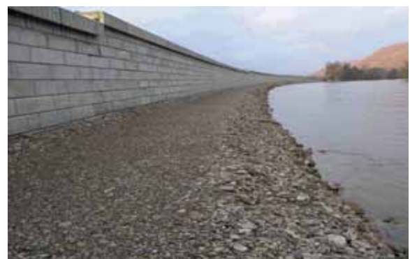
A TensarTech Marine System is well suited to aggressive coastal or tidal conditions such as harbour and river locations.
