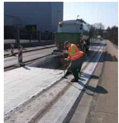
A simple overlap joint for Tensar Glasstex.
