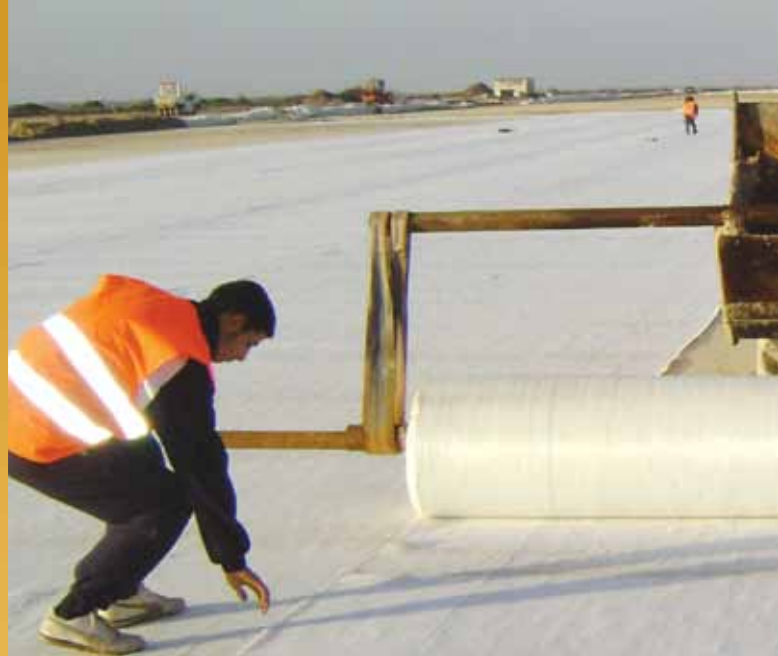
Tensar® Basetex™ installation at Oran airport in Algeria providing cost-effective installation and offering permanent stability to a critical load bearing surface.
