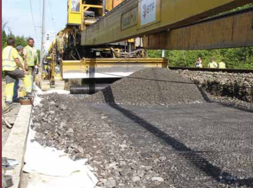
Tensor® TriAx® geogrids installed under the granular sub-ballast layer to increase bearing capacity (Belgium).
