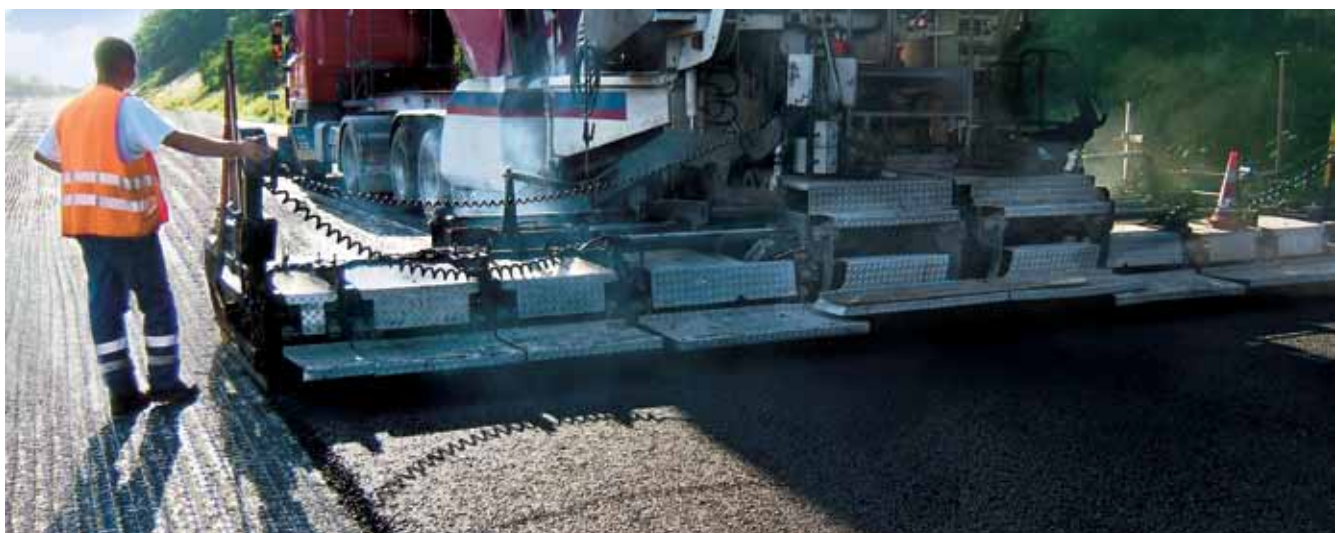
Paving takes place directly over the Tensar AR-G.
