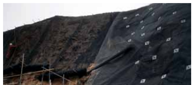
Tensar geogrids and mats are often used as a facing to soil-nailed slopes.
