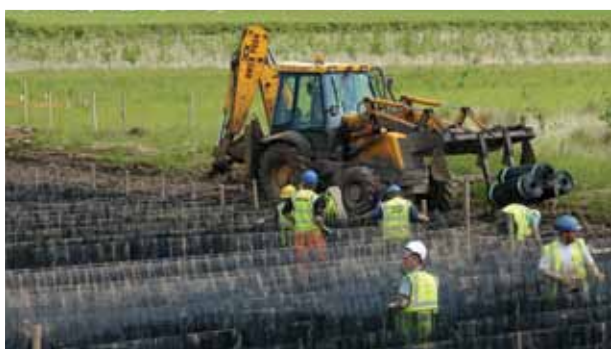
TensarTech™ Foundation Mattress System is used to control differential settlement over variable ground.
