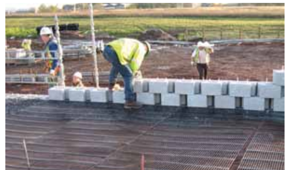
The modular block systems can be built without cranes or propping.
