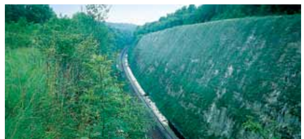
Geogrid used as face stabilisation.
