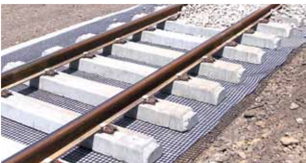
One method of installing Tensor geogrids below ballast prior to track lifting and tamping (Australia).
