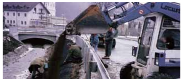
Tensar products are used to protect stream banks against erosion during periods of high velocity water flow.
