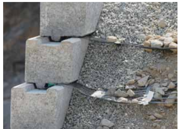
A feature common to all TensorTech Wall Systems is the high efficiency of the connection between geogrid and the chosen facing, in this case the TW1 Wall System.
